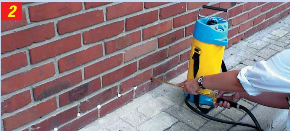
Fill boreholes with Aida® Injection Cream using a low pressure sprayer or cartridge gun.
