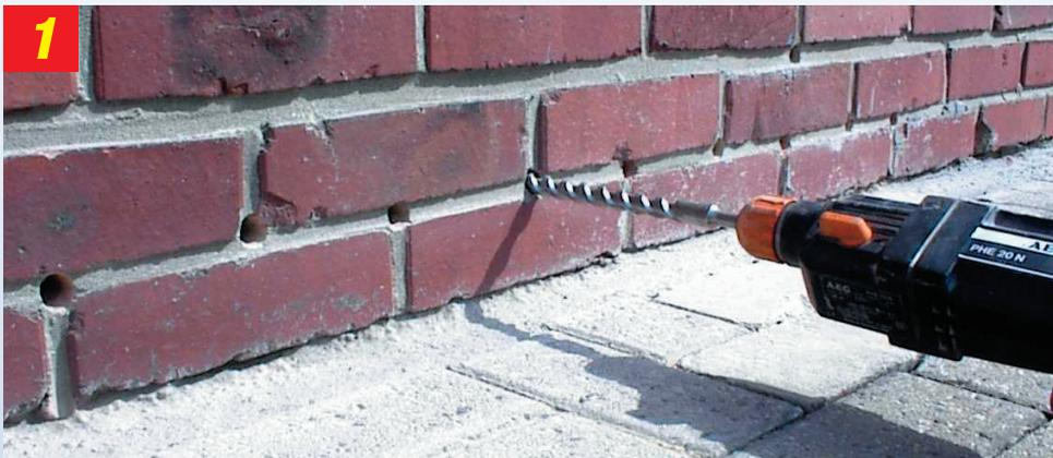
12 mm diameter holes drilled horizontally into the mortar joint at 120 mm centres and to a depth of 10 - 20 mm from the opposite face.
