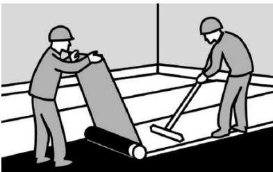
(Fig. 24) The covering strip that runs along the edge of the sheet must be removed to permit the sealing compound below to bond with the overlap of the adjacent sheet. As described above, align the neighbouring sheet and glue the two sheets together with a 100 mm overlap.
