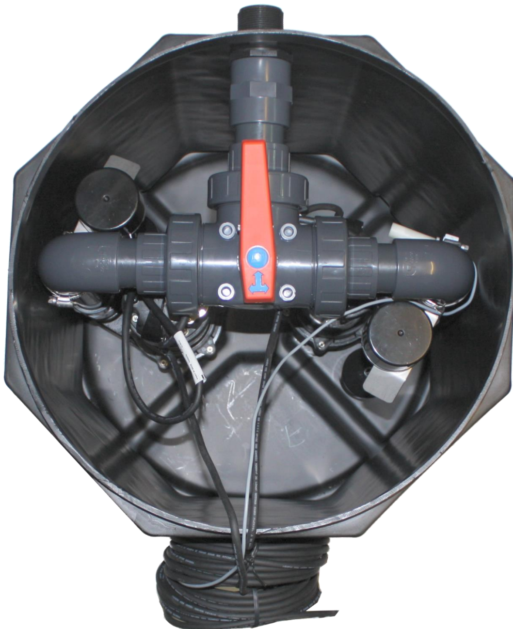
Fig 3 – dual pump set up.
